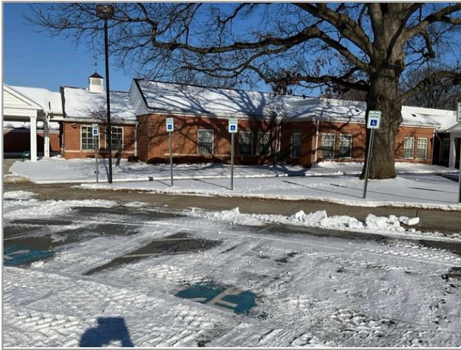
OVERVIEW OF ACCESSIBLE PARKING AREA
