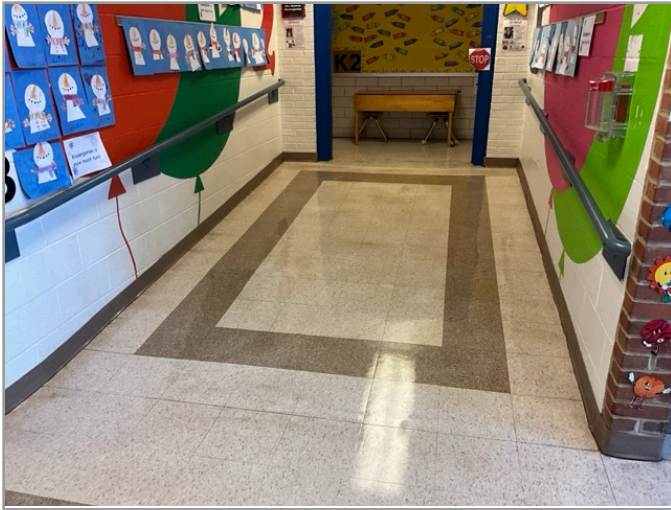
ACCESSIBLE INTERIOR RAMP
