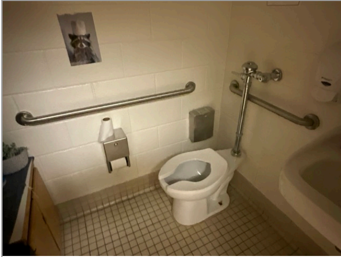
TOILET STALL OVERVIEW
